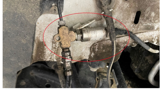
Fig. 5. Pressure sensor attached to the front right brake line.
